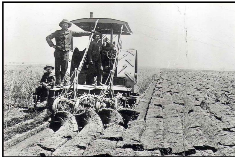
Fig. 1. Power machinery breaking virgin prairie sod in the early 20 th century. (Source: Western Development Museum, Saskatoon, SK).
